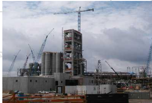
6000 TPD Preheater concrete tower
