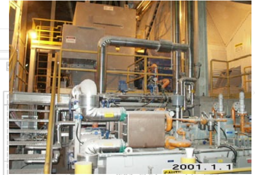
5000 hp preheater ID fan-synch motor with fluid clutch
