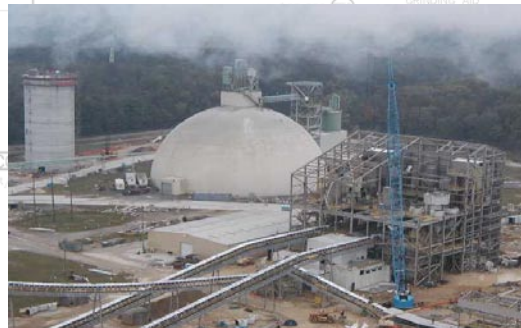
Cement storage dome
